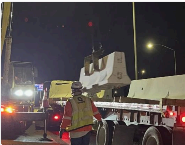
* using lifting holes
