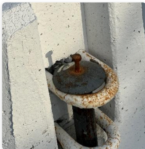
Safety Pin (Patent Pending) and example of a pulling device
