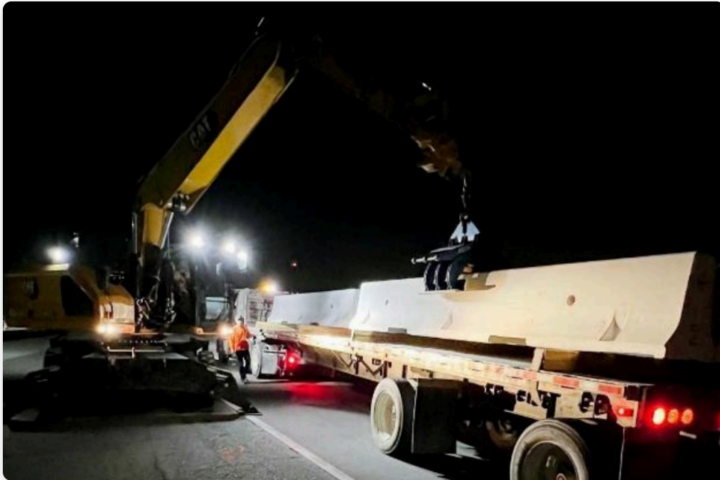
* using the lifting clamp
